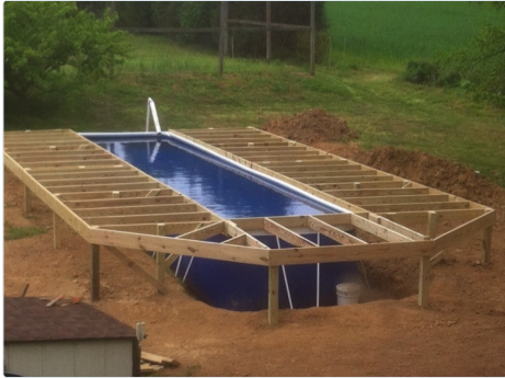
Pool filled, joists complete.
