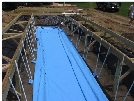
Pool laid out in the space, ready to be erected.
