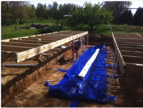
Deck framing out, liner going in.
