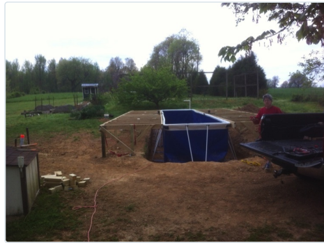
Assembled pool, finishing the deck supports.
