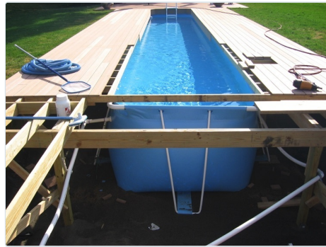
Liner full, deck work in process.
