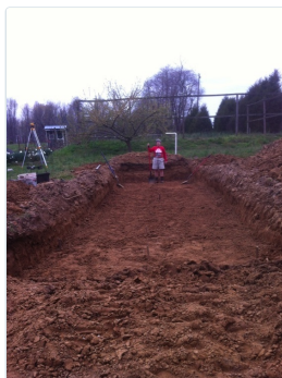
Leveling the ground.
