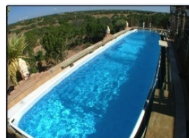
The finished terrace from above.
