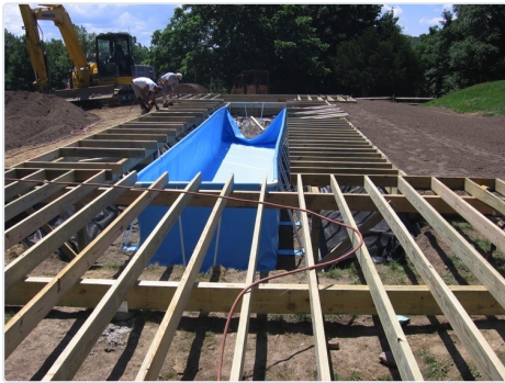
Deck framed and the pool erected.
