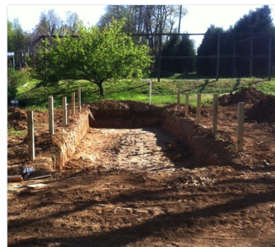
Preparing for the deck supports.
