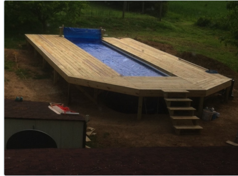
Deck surface in place.
