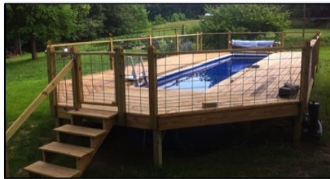
The finished deck with railing and steps.
