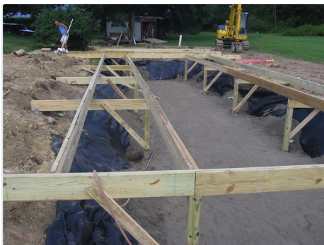
Hole dug and deck framework built.
