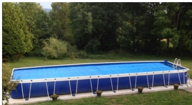
The same pool from the side — a paver under each vertical support.
