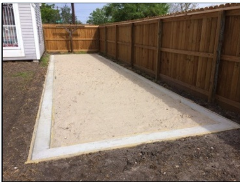
A concrete perimeter with the interior filled with sand.
