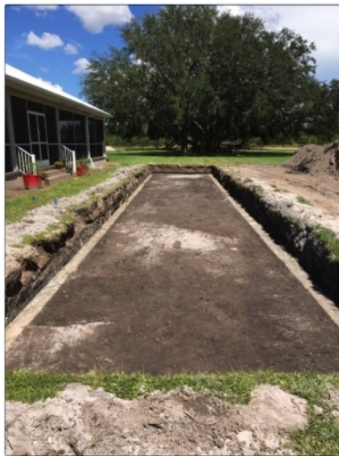
The hole freshly dug.
