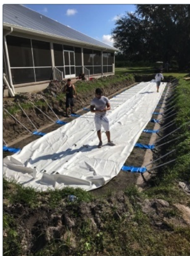
Laying the liner out in the hole.
